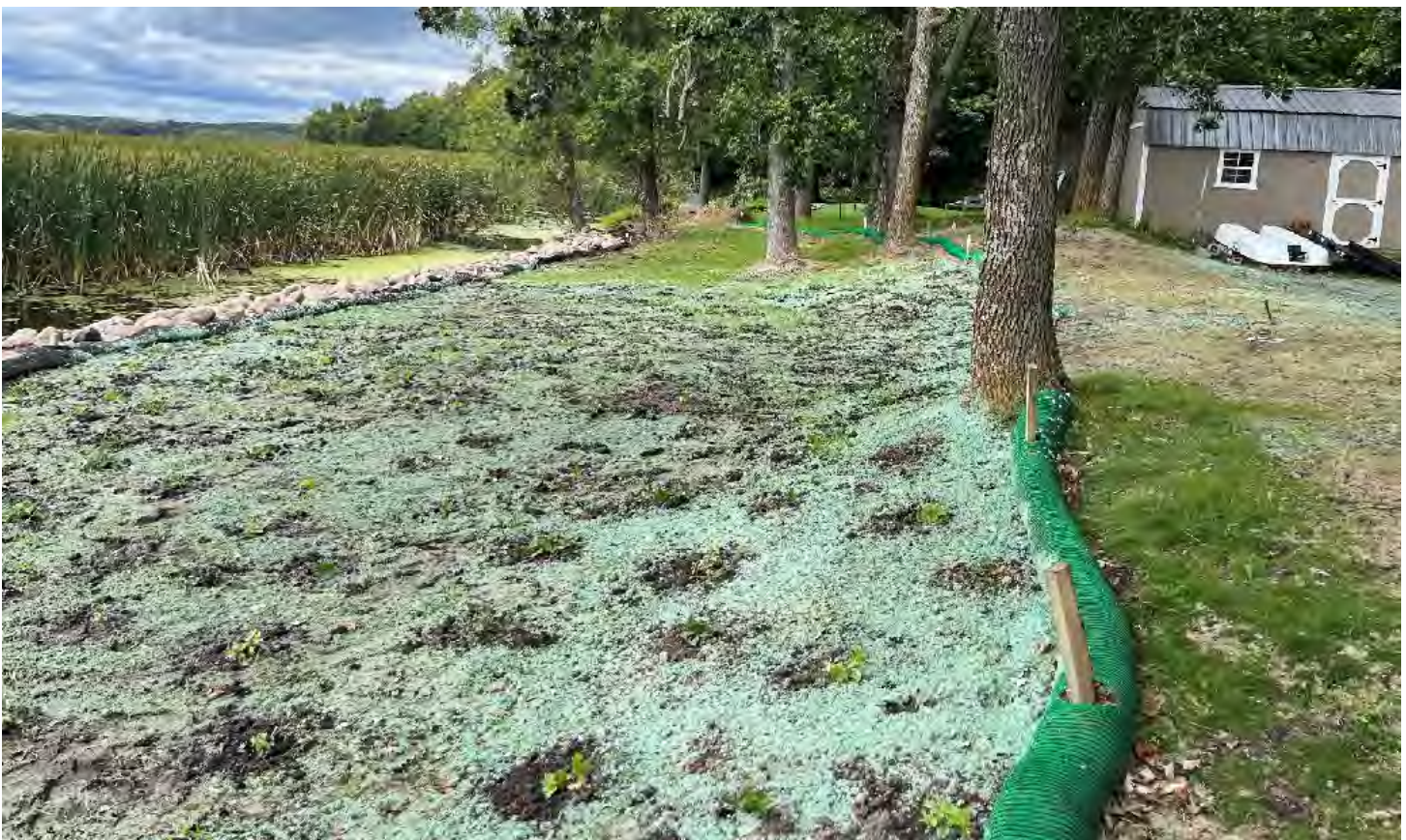
Buffer area completed (Plugs planted and partially non-native wildflower seed mix planted with hydro mulch)
