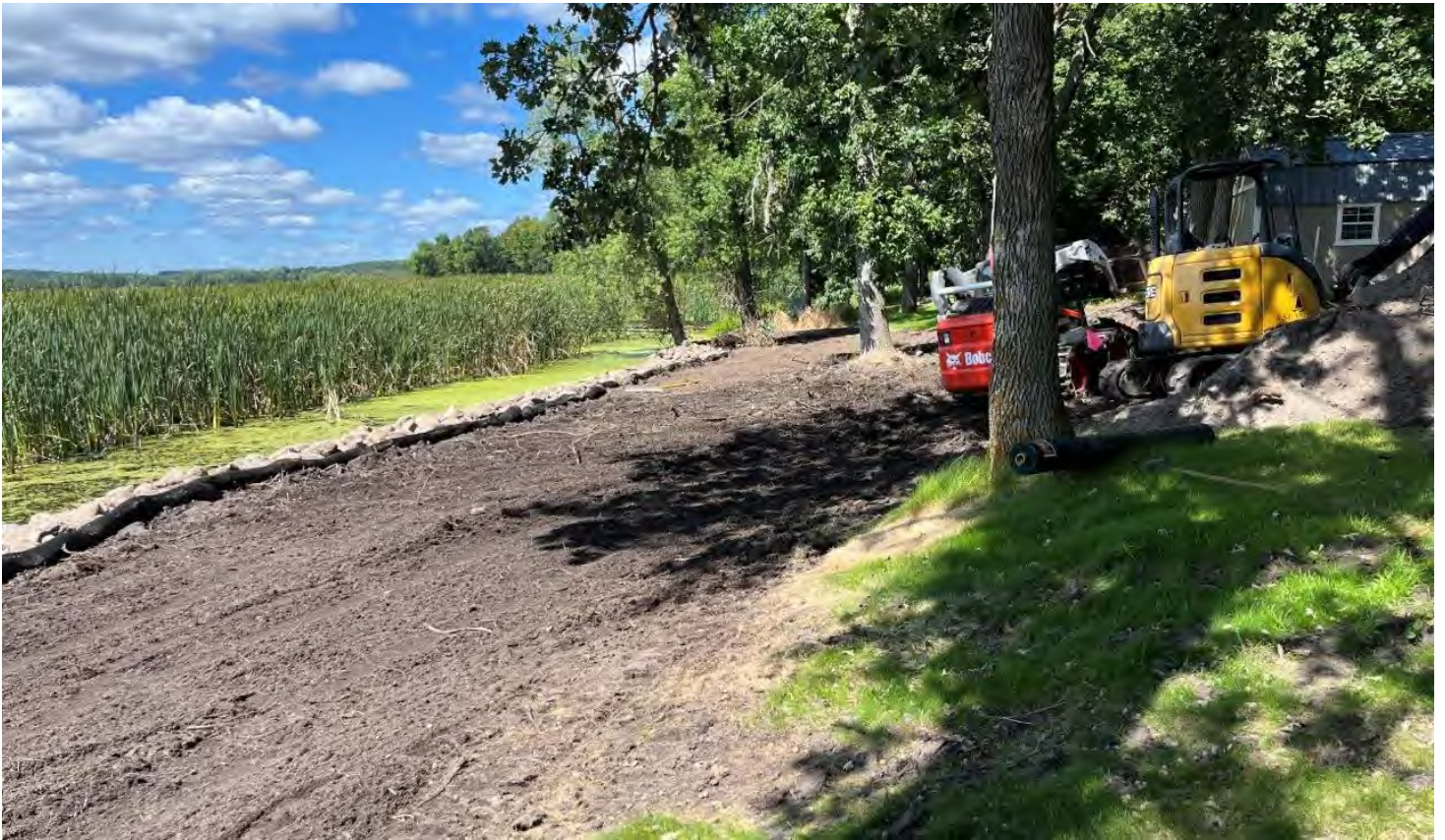
Rock installed & contractor prepping buffer area for planting of seed and plant plugs
